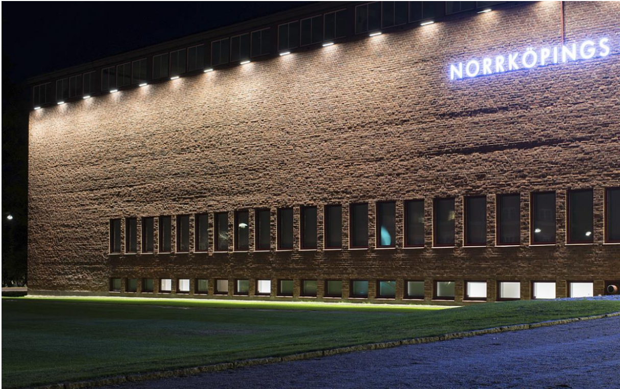
Figure 5. Advertising lighting ( https://www.erco.com/en/projects/public/correctly-illuminating-facades-7... )
