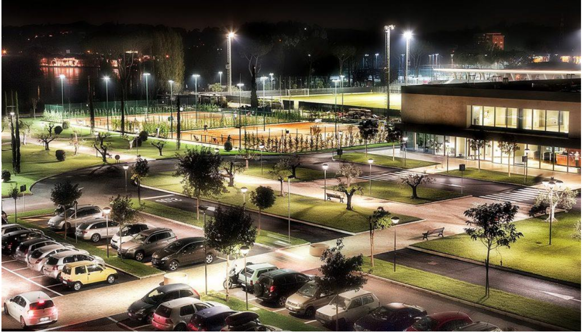
Figure 3. Outdoor parking lot lighting ( https://www.aydinlatma.org/acik-otopark-aydinlatmasi-nasil-yapilir.html )
