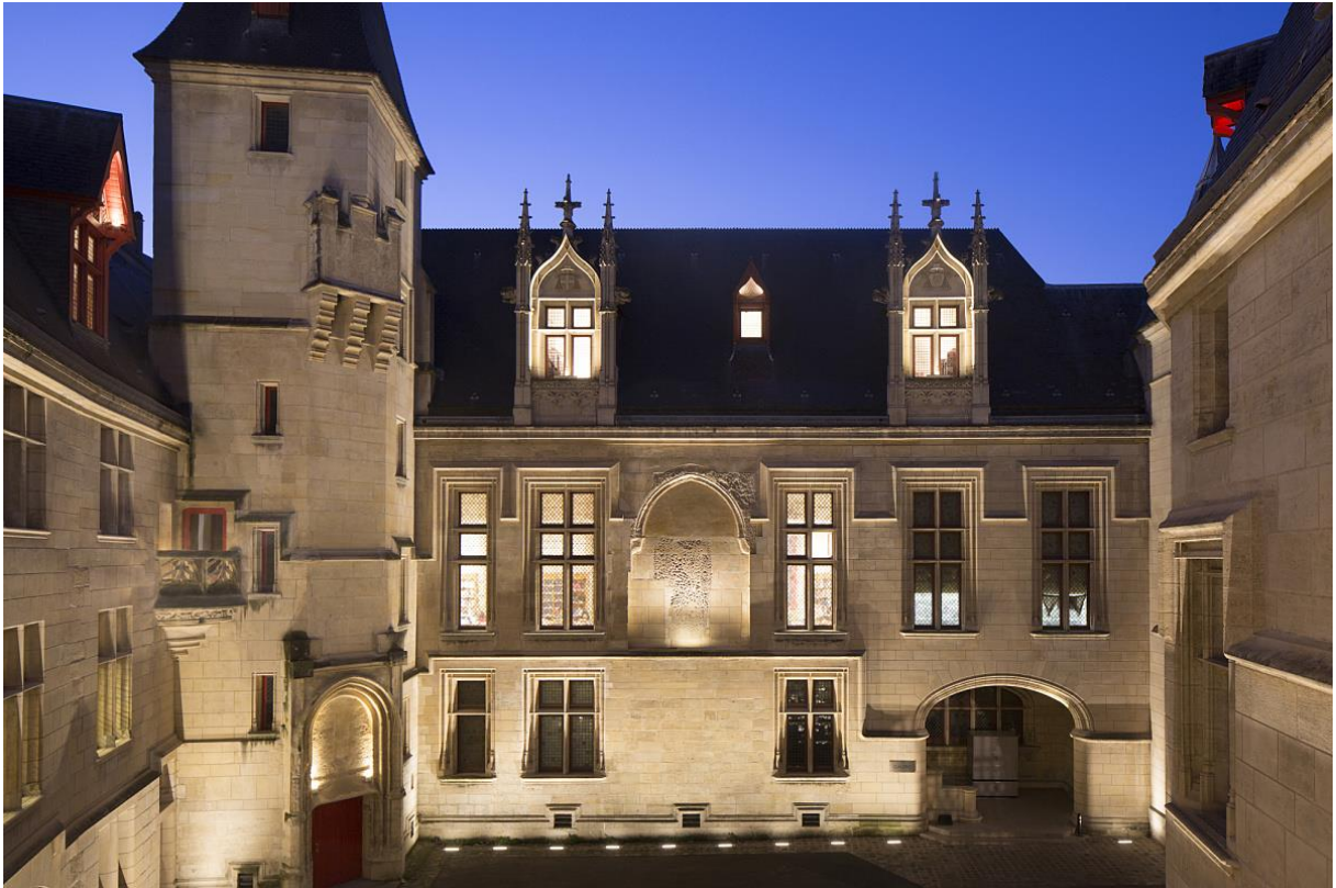
Figure 4. Facade lighting ( https://www.erco.com/en/projects/public/correctly-illuminating-facades-7... )
