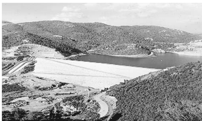
Fig. 2 General view of the Tahtalı dam site
