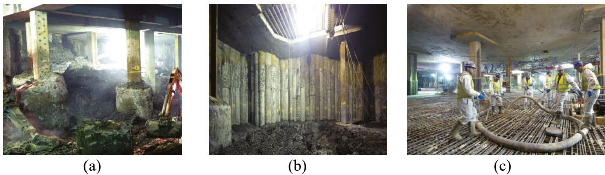
Figure 3. (a-b) Southwark Tower basement views, (c) concrete pouring process (URL-9)
